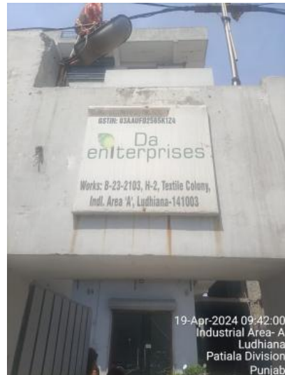
Facility name board.jpeg
